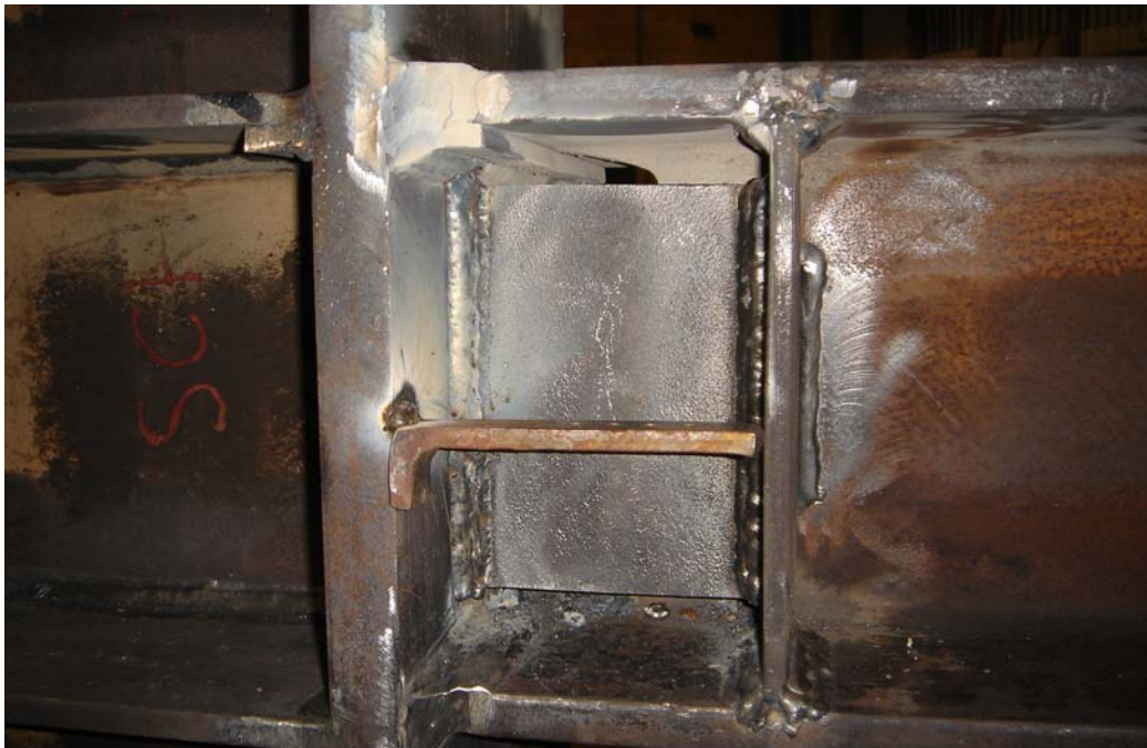
Figure 2.45: Specimen AISC-7 after Completion of Fabrication – Backside of Link
