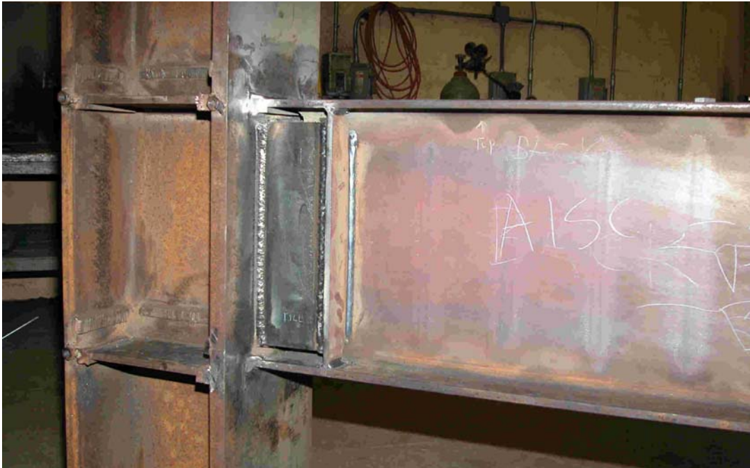
Figure 2.32: Specimen AISC-5 after Completion of Fabrication – Backside of Link
