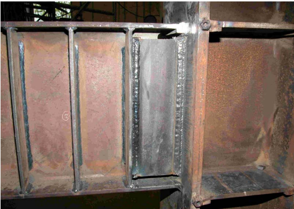
Figure 2.31: Specimen AISC-5 – Link-to-Column Connection Region – Frontside of Link
