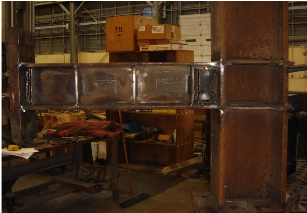
Figure 2.40: Overall View of Specimen AISC-6 after Completion of Fabrication
