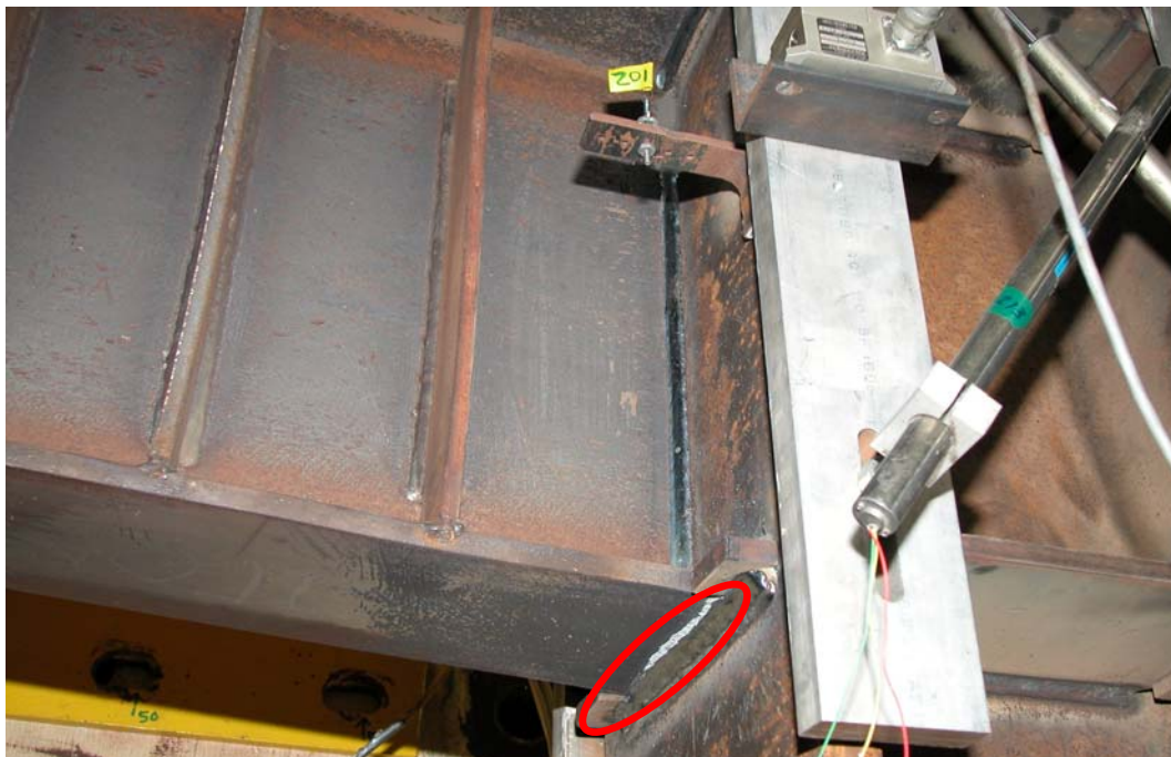
Figure 3.12: AISC-3 – Fracture of the Bottom Link Flange during loading cycle at \gamma = - 0.09 rad
