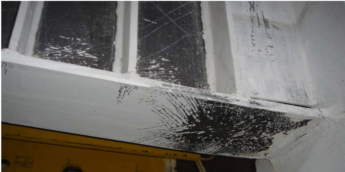
Figure 3.55: AISC-8 Link Bottom Flange at the Link-to-Column Connection after Loading Cycle of \gamma = \pm 0.07 rad (Last full loading cycle prior to failure)
