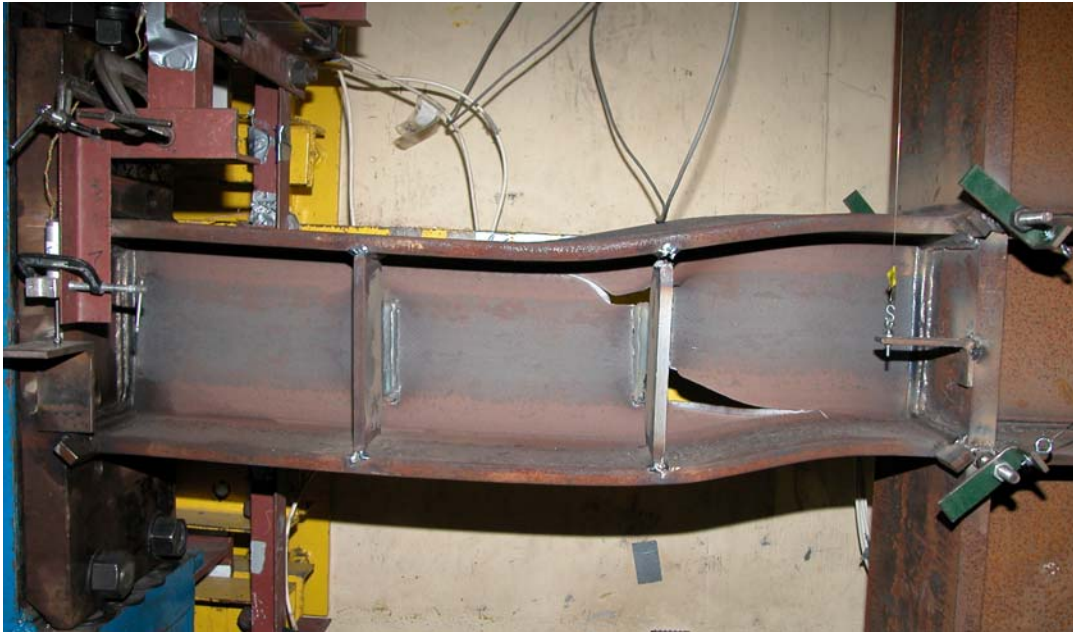
Figure 3.19: Failure of Specimen AISC-4 during loading cycle of \gamma = + 0.13 rad
