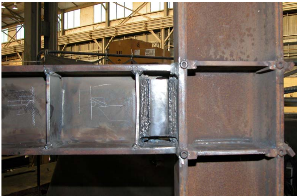
Figure 2.41: Specimen AISC-6 – Link-to-Column Connection Region – Frontside of Link
