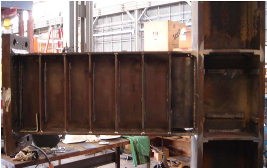
Figure 2.33: Overall View of Specimen AISC-8 after Completion of Fabrication
